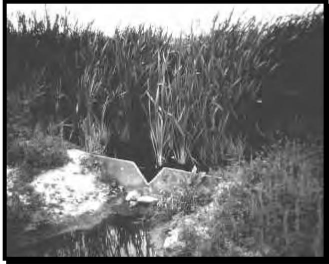
**Figure 11: Simple V-notch Weir**
